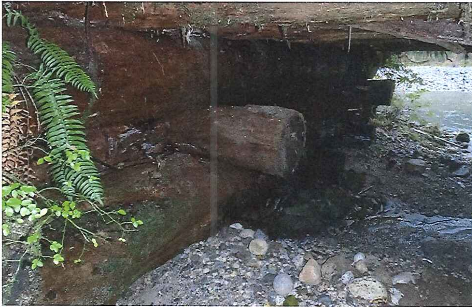
CK2264 Left Abutment
